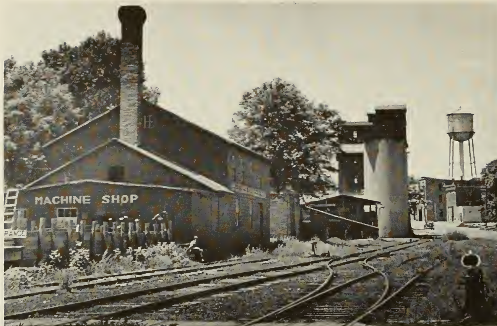
Libertyville's first electric power house . . . now known as the Laycock Machine Shop
